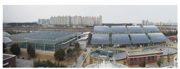
Figure 17: Renewable energy facilities of the Gangneung Wastewater Treatment Plant
