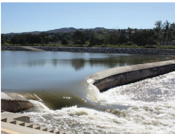
PHOTOGRAPH 3.2. Inflatable Rubber Dams Used to Maximize Groundwater Infiltration, Orange County, CA
