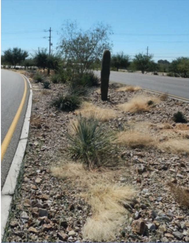
a. Xeriscaping to capture and infiltrate stormwater
