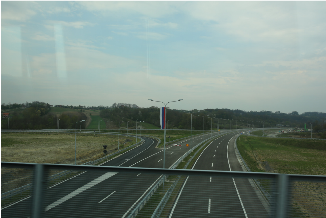
Photo I: Banja Luka-Doboj highway "9 January"
